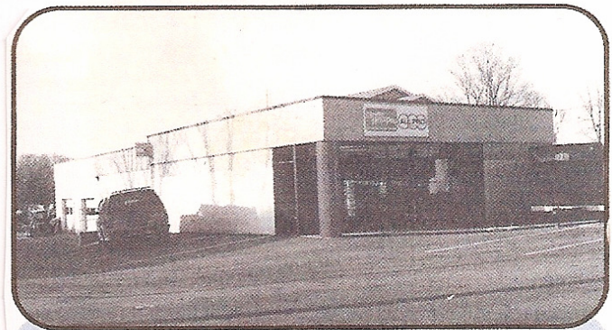
All-Pro headquarters in Mechanicsburg, Pennsylvania: 4 Bays and 5,000 sq. ft. of work area.
